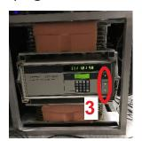
a) Check **USV** for GPS (green LED on) b) Check **USV** for 10 MHz (green LED on)
